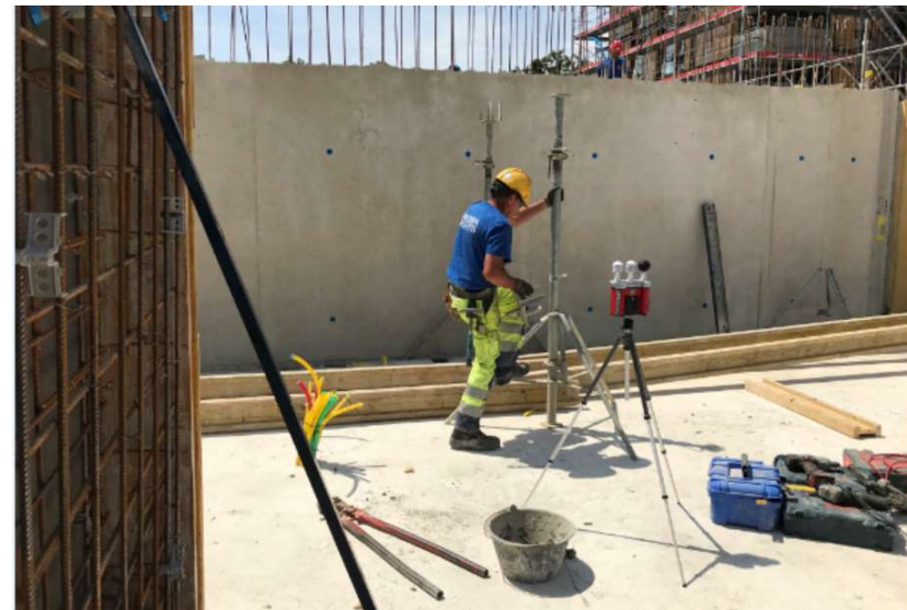
Preparation of slab formwork base
